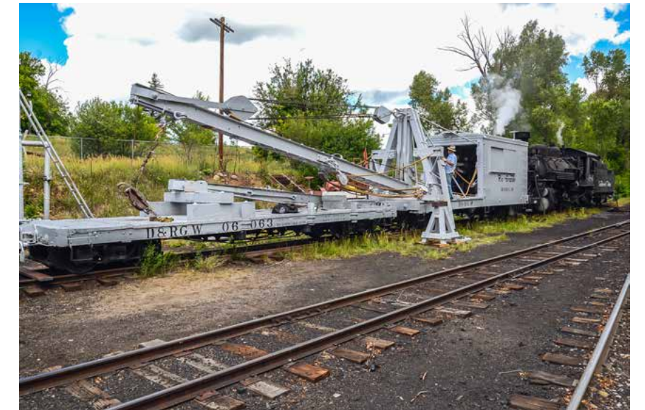
Testing the rigging and working the lift. Exciting stuff for the team after all the work they put into this project.
