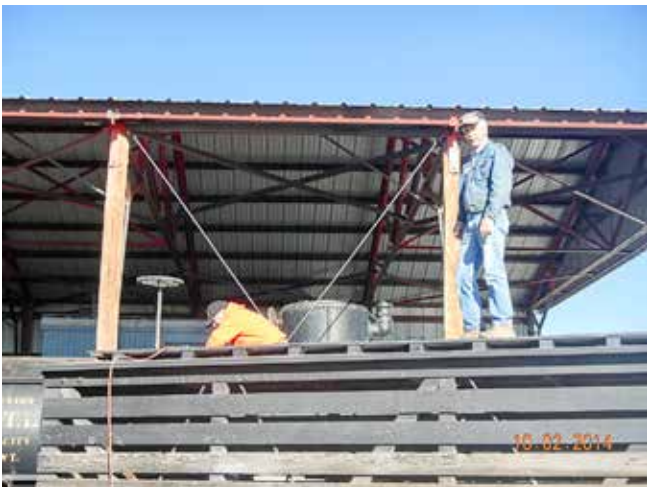
Doug Joslyn and Kevin Corwin testing replaced roof walk on 5995.
