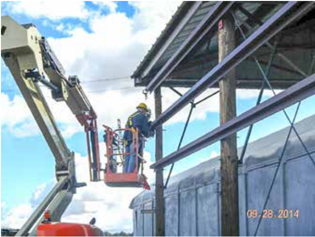
Chuck Dueker and Jim McGee prep for car shelter siding installation
