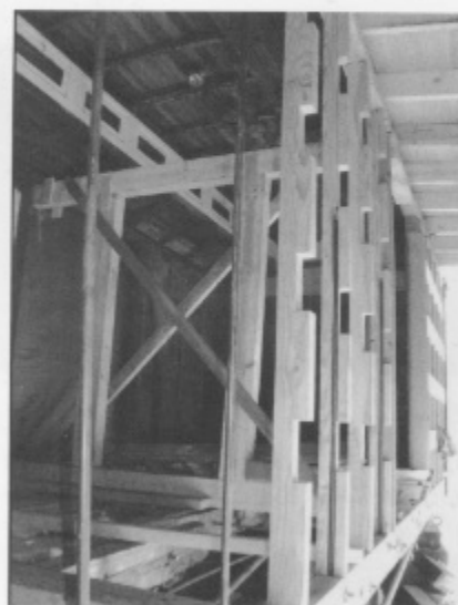
New right side vertical supports in place A end.
