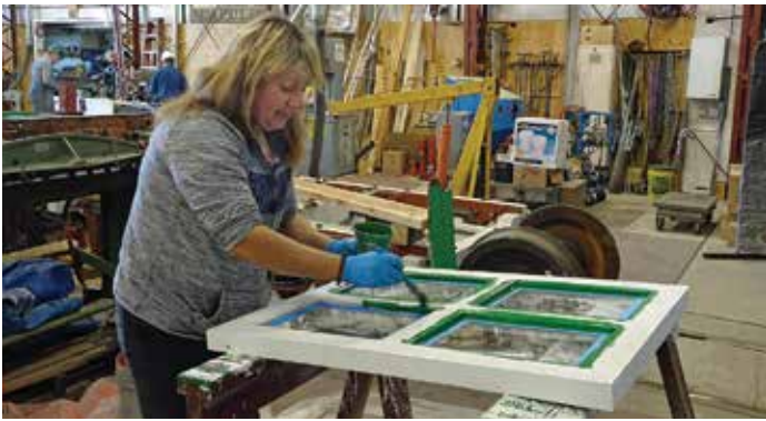
New windows and doors were built and painted.
