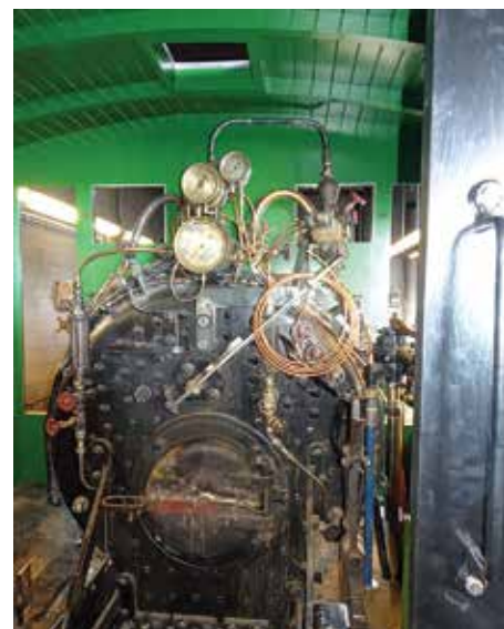
The cab's interior and controls are restored and inspected.
