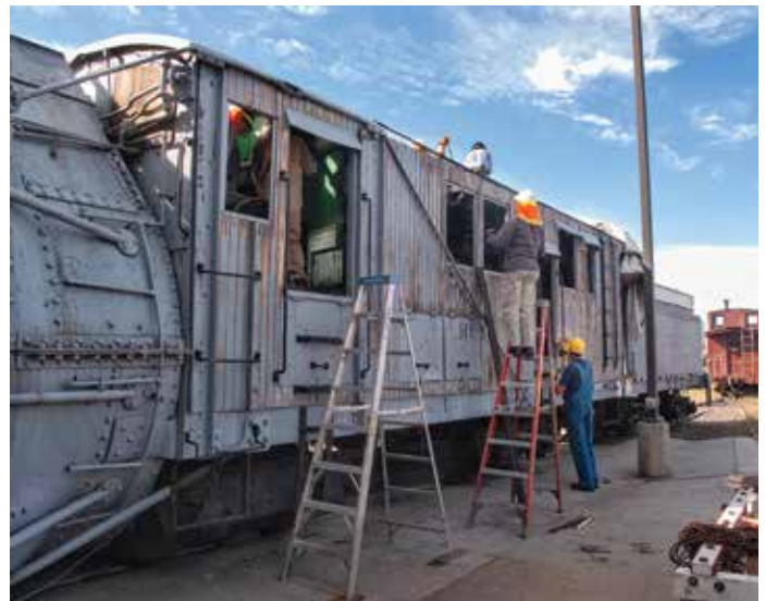
Friends restore the exterior and prepare to paint. Photo by Chris James
