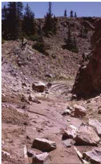
Some parts of the right-of-way needed more work than others.
