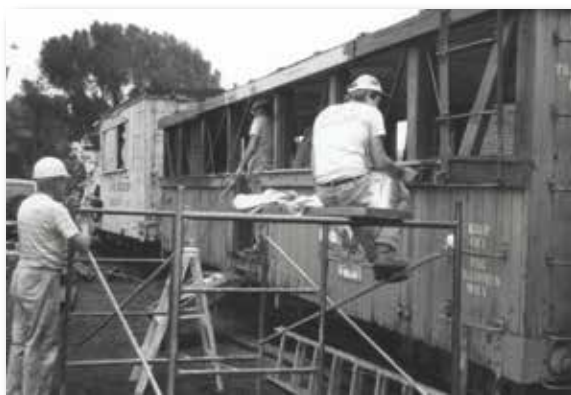
Boxcars quickly are converted into passenger cars.
