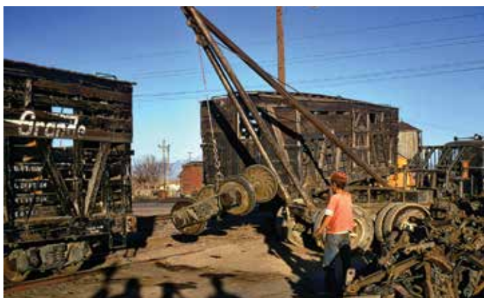
Scrapping D&RG livestock cars in Alamosa, November 28, 1967. With the metal parts salvaged, most of the wooden cars were burned. Photo by Ernie Robart FCTS ERNG19671118-0220
