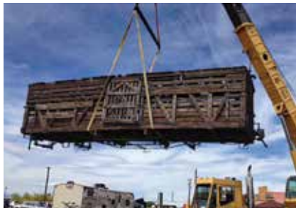
34-foot Stock Car 9559 is raised to be placed upon a set of trucks and to begin restoration. Photo by Dan Pyzel
