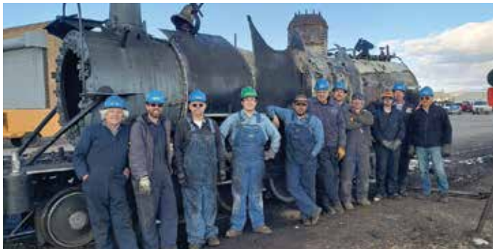
The inspection began with the removal of the boiler jacket and cab. The DRHS and C&TS shop crew at Antonito.
