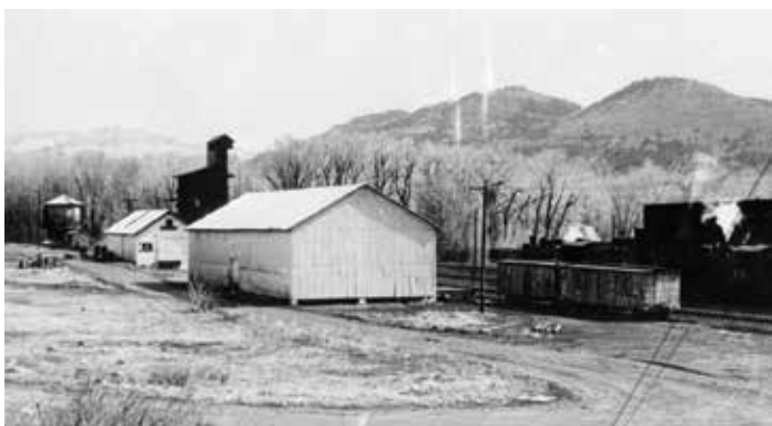
Chama's wool warehouse in the early 1950s. It was situated in what is now part of the depot parking lot. FCTS RD010-025
