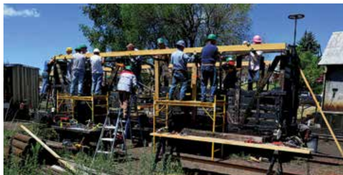
When it came to restoring Stock Car 5991, many hands made light work placing a roof beam. Here, a dozen or more Friends volunteers join Bill's team in the Chama yard, Session C, 2019. Photo by Dave Jenkins
