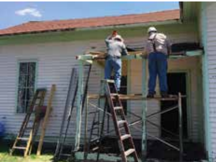
Repairs at the Sublette Section House.
