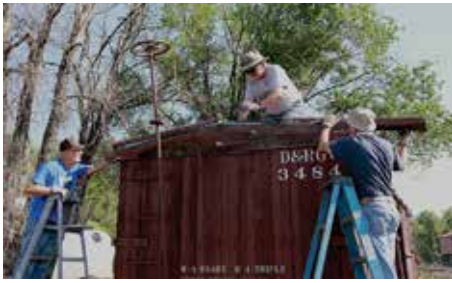
Roof repairs on Box Car 3484.
