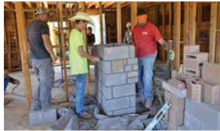
A new chimney in the Car Inspector's House, both inside...
