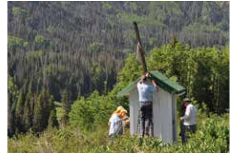
Telegraph booths got some needed repairs.
