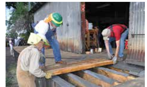
Repairing the deck at the Carpentry Shop.
