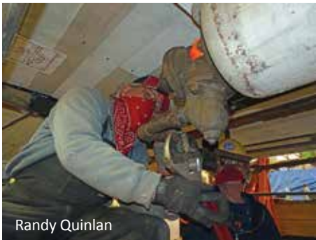
The triple valve was cleaned, inspected and mounted to the air reservoir.
