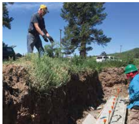
Foundation for the Chama Storage Building.
