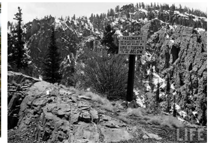
MP 315.328 Sign at Toltec Tunnel Circa April 1950 Photographer Wallace Kirkland
