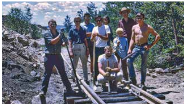
Ernie (L) helps repair track in the Narrows, 1970 FCTS Collection
