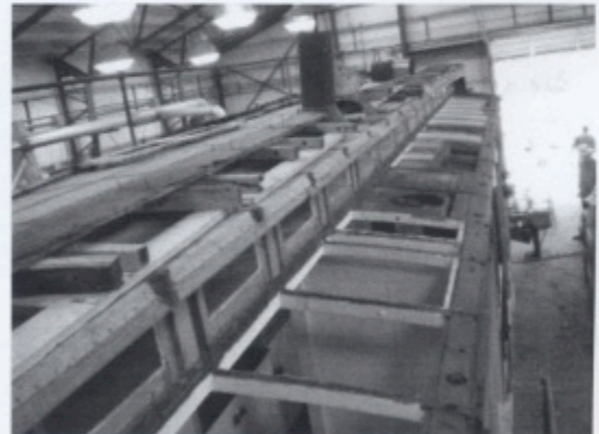
Rotten wood under the tin has been removed.
