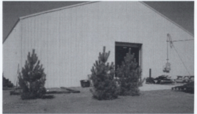
Three trees were planted at the northeast corner of the CRF.
