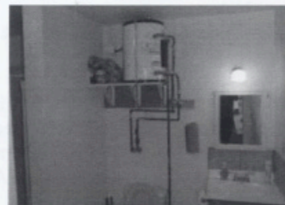
Marshall Smith and Bob McCain made short work of this installation.
