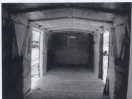
New 3/4" T&G OSB sub-floor installed.
