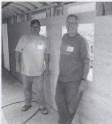
Exterior siding and interior sheathing crew Kevin Sherrow & Barry Morris
