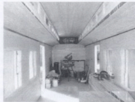
Interior B end - RPO end.
