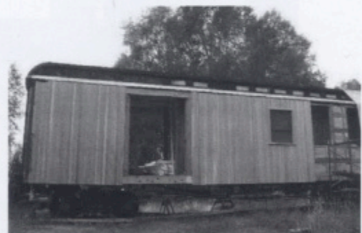
First window installed.
