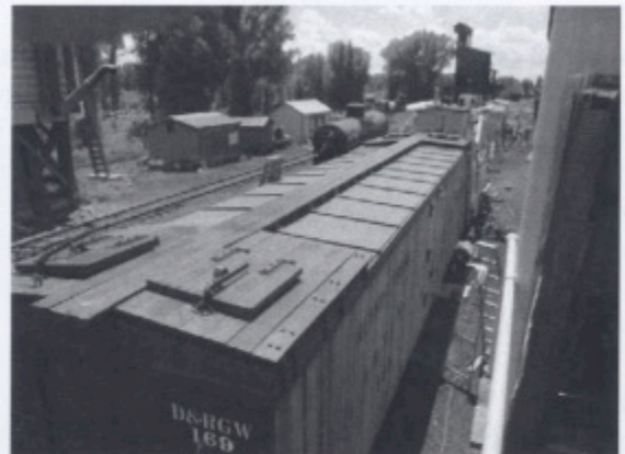
Hatches and catwalks newly hand painted.
