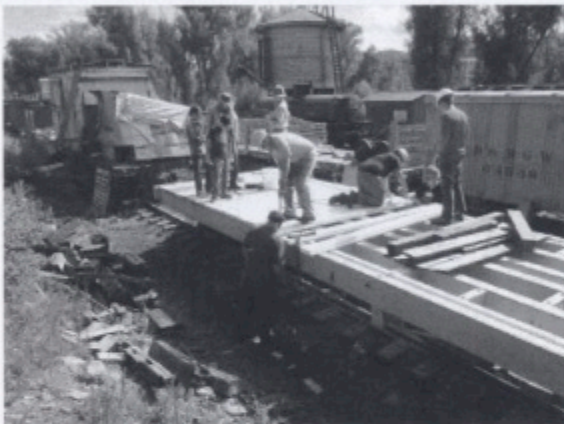
The whole crew including two Boy Scouts installing the ship lap deck planks.
