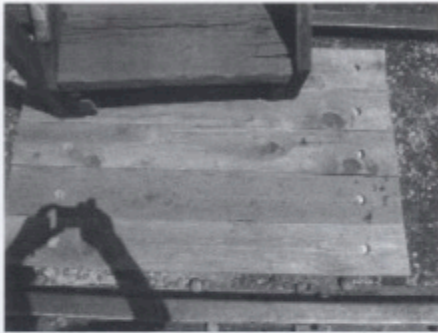
Wooden platform installed by the fastener car steps.
