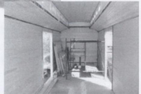
Interior A end - Baggage end.
