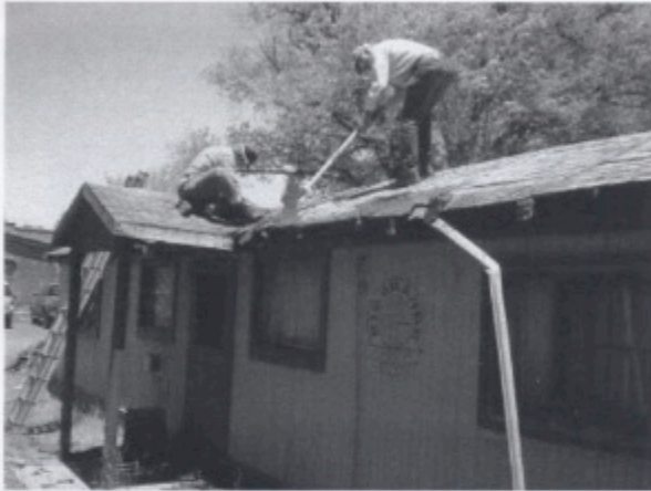
Fred Morton and Ron Horesji removing old roofing material.
